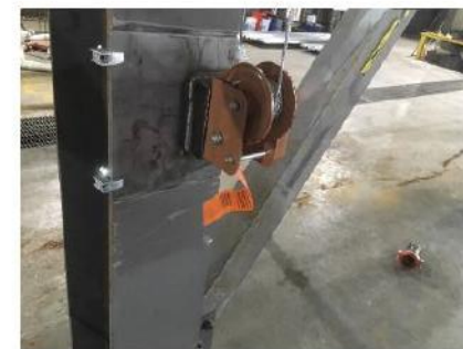
Figure 2-5: Crankshaft for smoke vent activation.
